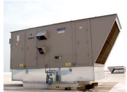
The SEMCO Revolution® natural gas desiccant dehumidification/air conditioning unit delivers comfort and savings at Lowe's.
